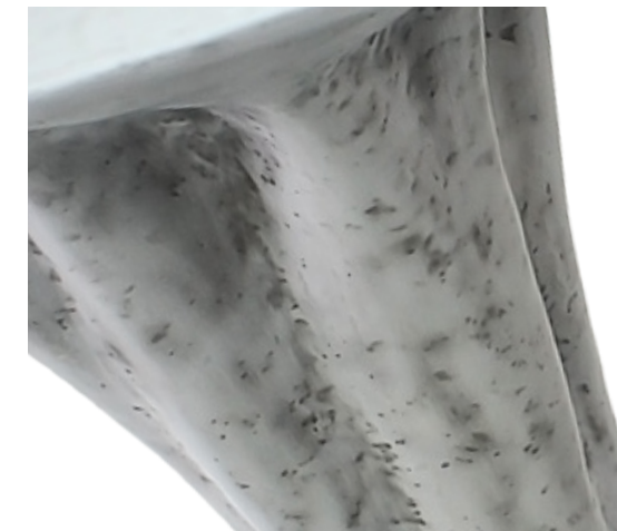
Aged concrete finish.
